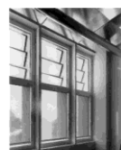
Figura 107.1 Daylight system for vertical windows Adjustable prismatic panels on exterior with diffracting prisms/louvers integrated into the window
